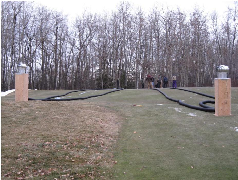
Installation of passive ventilation using whirlybird roof turbine to produce continual airflow
